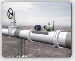
Flow Control Collect Flow Data with intrinsically safe Wireless Nodes that provide battery power to the radio and transmitter (ATEX)
